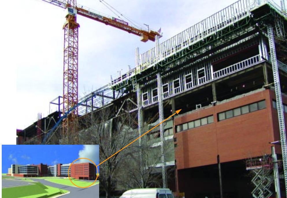
Three stories were added on top of an existing four-story wing.
